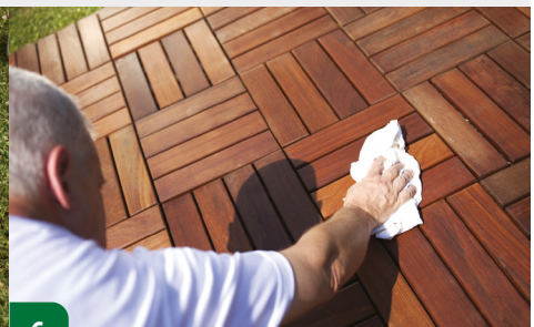
6 After about 10 minutes remove any excess product with a cloth. Repeat the treatment if necessary, allowing sufficient drying time between coats.
